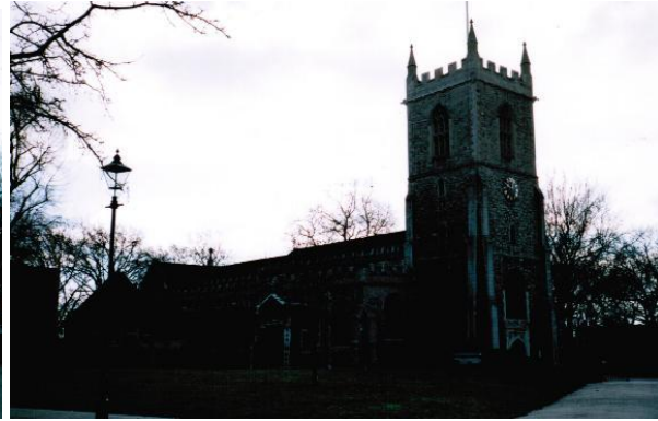
Two months later, and the scaffolding is all gone, and the work complete, at St. Dunstan's Stepney. March 2006.
