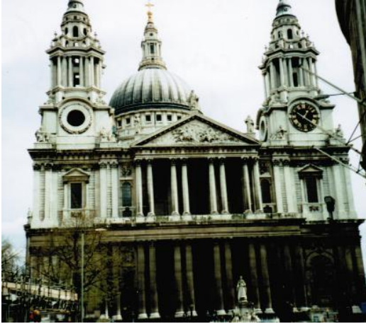
St. Paul's Cathedral, London, April 2001 on Gavin's first trip to London. Note the black soot on the lower part.
