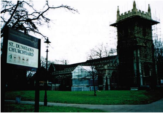
St. Dunstan's Stepney, London, E1, with some repair work being undertaken on its bell tower and elsewhere. January 2006.
