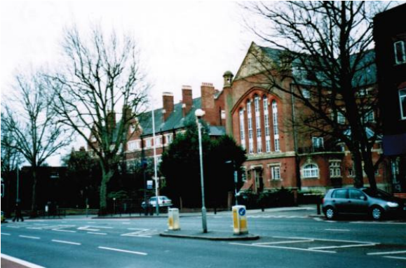
Old New College building (1924-1977) after reconstruction work. Dec. 2005 / Jan. 2006.
