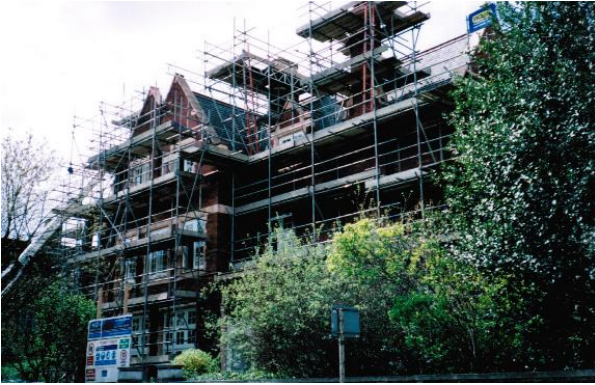
New College, London University (1924-1977), building being renovated for French College (on a 23 year lease). Corner of Parsifal Road & Finchley Road in West Hampstead, London, NW3. April 2004.
